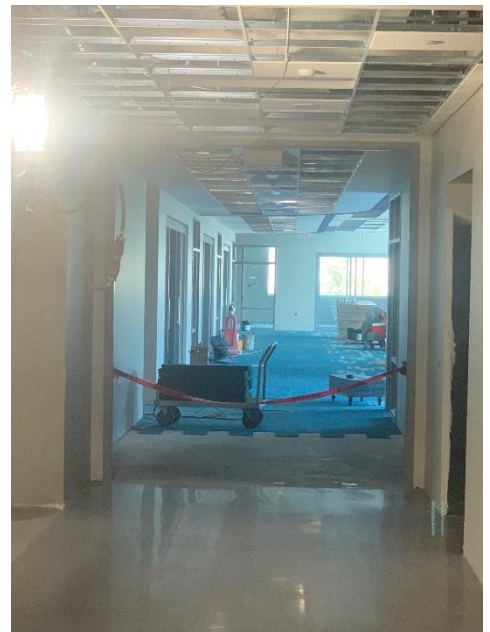
28. Area 3&4 – Terrazzo floor is getting sealed in second floor flex café and carpet install in gradewing area in progress.
